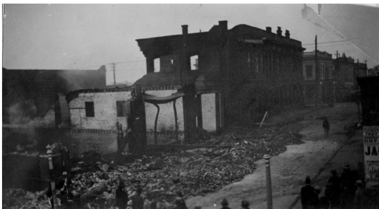
1934 fire damage; southwest view across Church Street with Carroll Building in background.
