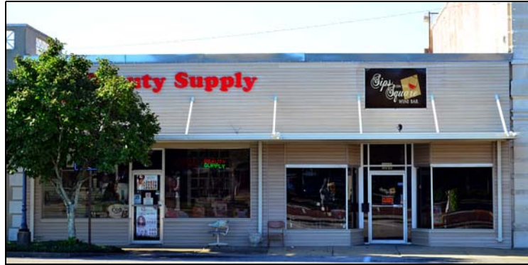
Figure 4.21. South elevation at 18-24 and 18-25.
