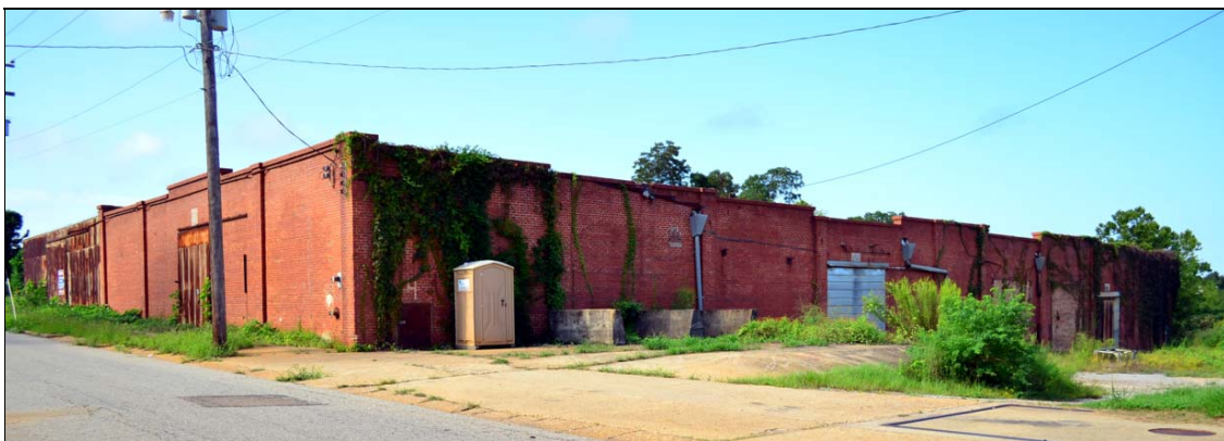
Figure 4.75. Sessions Warehouse East, northeast oblique.
