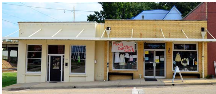
Figure 4.50. Buildings 9-51a and 9-51b (right to left), north elevation.
