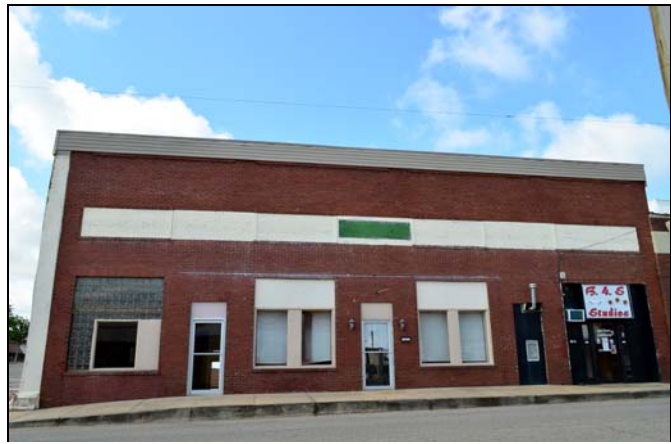
Figure 4.9. North elevation at O’Neil Motor Company Annex.
