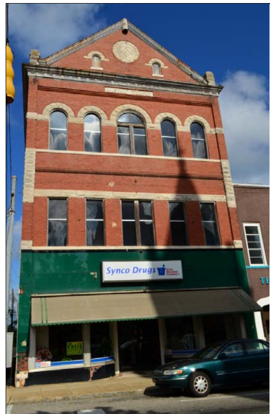
Figure 4.37. Masonic Building, east elevation.
