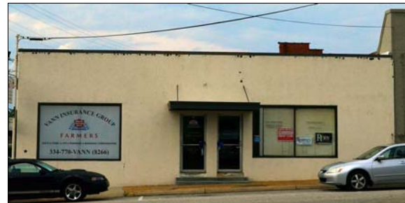
Figure 4.26. Vann Insurance Building, south elevation.
