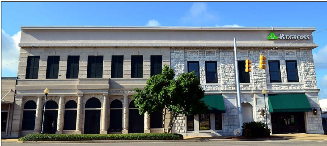
Figure 4.22. North elevation at F&M building (left) and Telephone Exchange building
