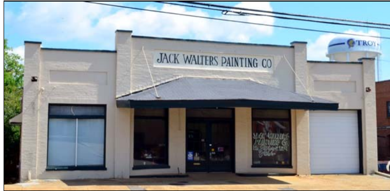
Figure 4.56. Walters Building, south elevation.
