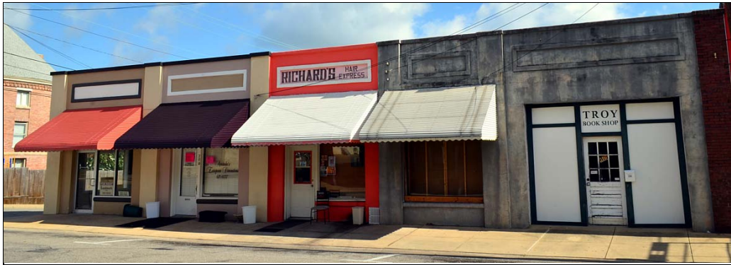
Figure 4.43. 7-11.4a, 11.4b, 11.2, and 11 (left to right), south elevations.
