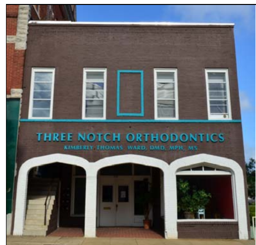
Figure 4.40. 5-14, Ward Building, east elevation.
