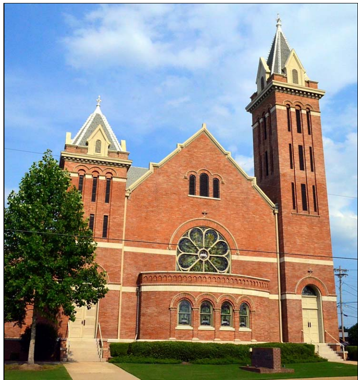
Figure 4.41. Methodist Church, west elevation.
