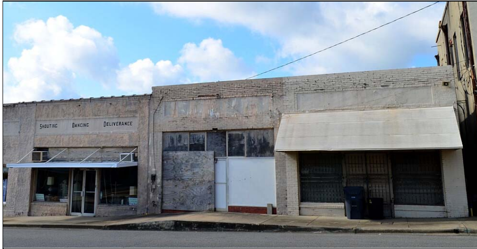
Figure 4.14. North elevations at 14-60a, 14-60b, and 14-59a (right to left).
