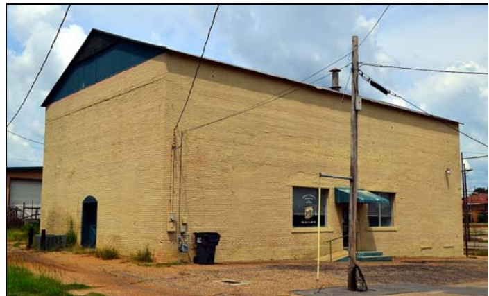
Figure 4.60. Co-op Gin Building, southeast oblique.
