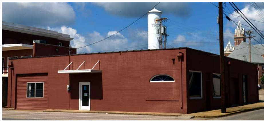
Figure 4.47. Johnson Center Annex, northeast oblique.
