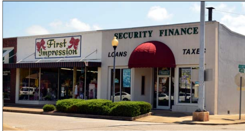
Figure 4.13. First Impression and Security Finance buildings, west elevation.
