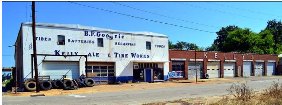
Figure 4.74. Kelly's Tire Building, south elevation.
