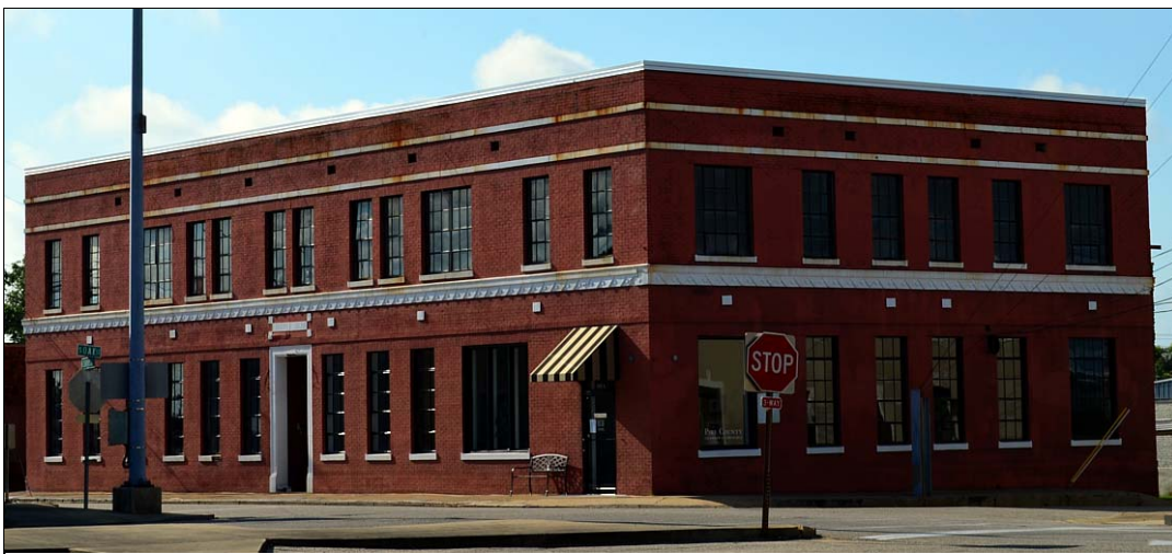
Figure 4.17. Carroll Building, northwest oblique.
