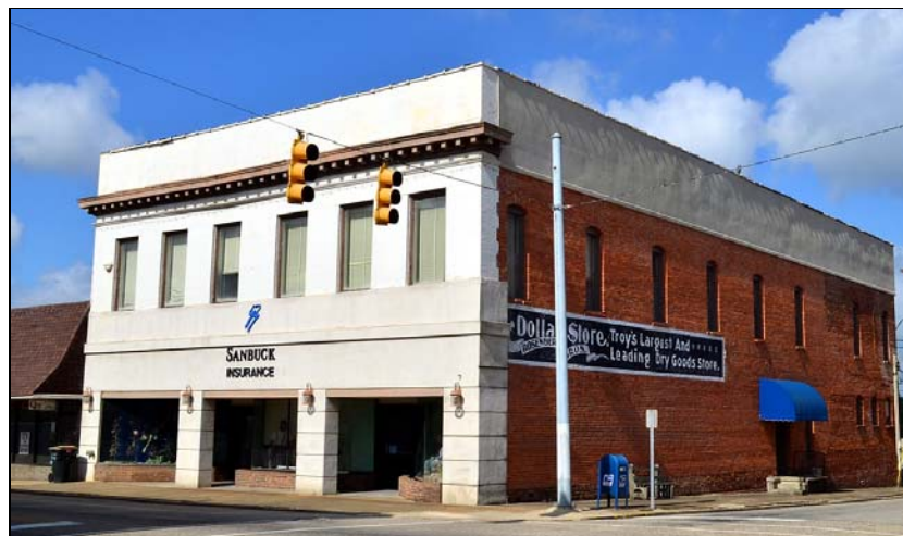
Figure 4.23. Rosenberg Building, northeast oblique.
