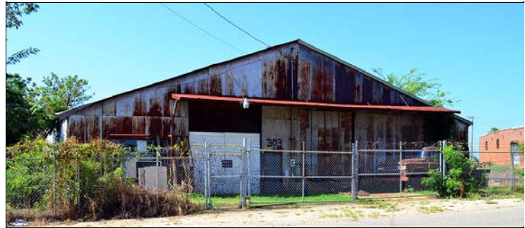
Figure 4.72. Carroll Warehouse No. 3, north elevation.
