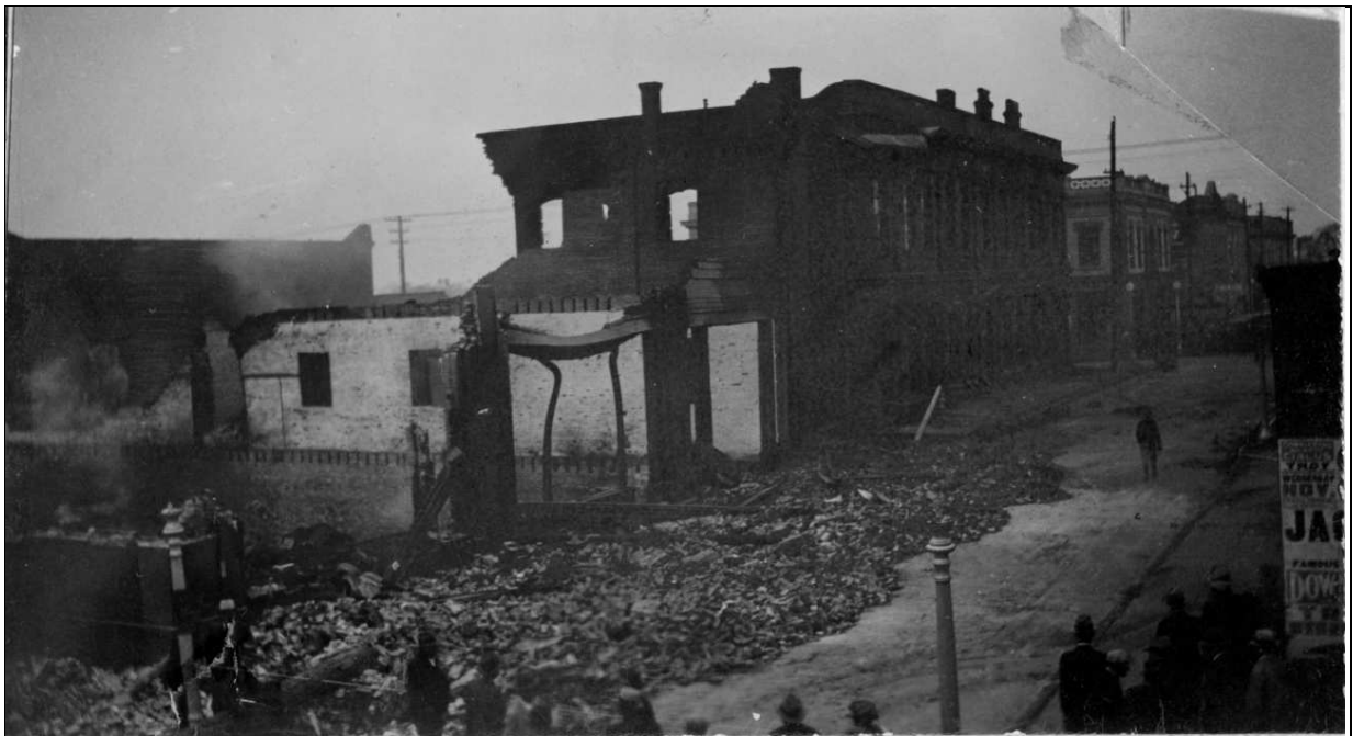
Figure 2.3. 1934 fire damage; southwest view across Church Street with Carroll Building in background.
