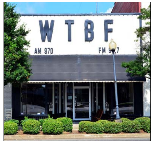
Figure 4.30. WTBF Building, east elevation.
