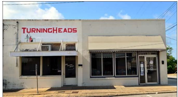
Figure 4.68. Buildings 22-43 and 22-42a, north elevation (right to left).
