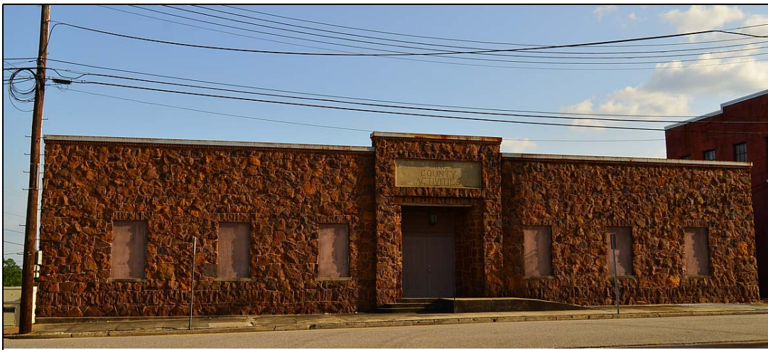
Figure 4.18. North elevation at the Rock Building.
