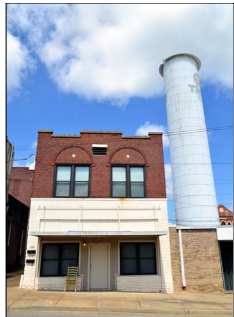
Figure 4.7. West view of water tower and 11-37 east elevation.
