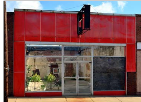
Figure 4.44. Building 7-10, south elevation.
