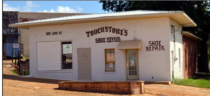
Figure 4.67. Touchstone's Shoe Repair, southwest elevation.
