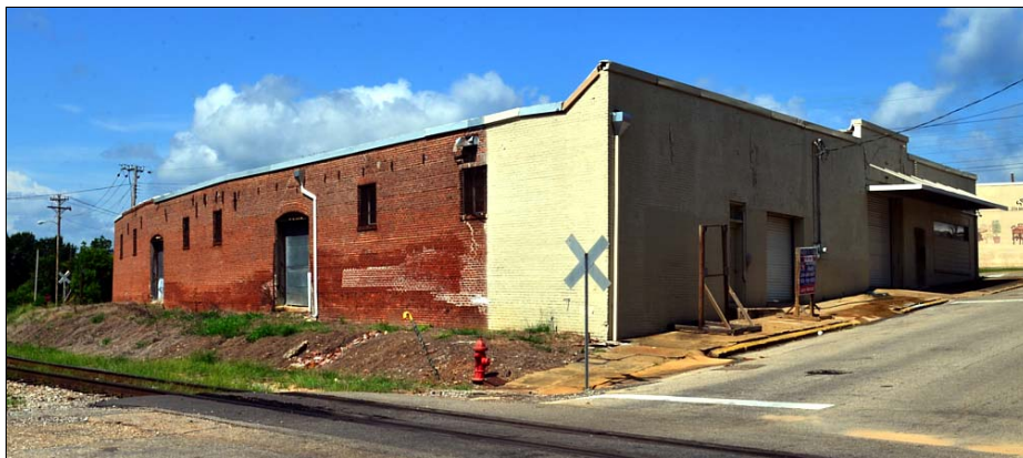
Figure 4.71. Seals Warehouse, northeast oblique.
