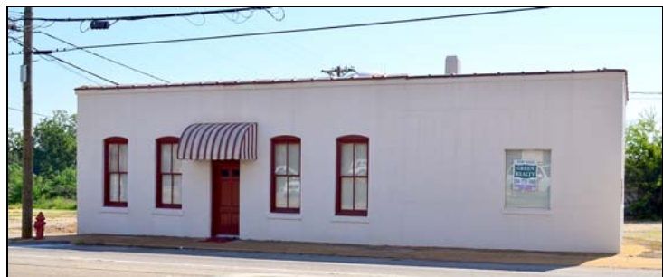
Figure 4.62. Building 4-5.1, west elevation.
