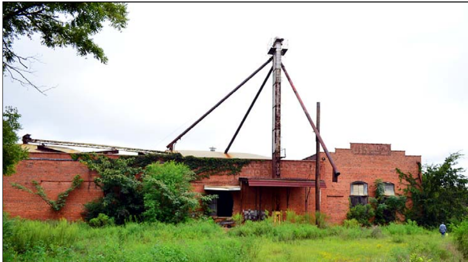
Figure 4.76. Alabama Warehouse No. 2, south elevation.
