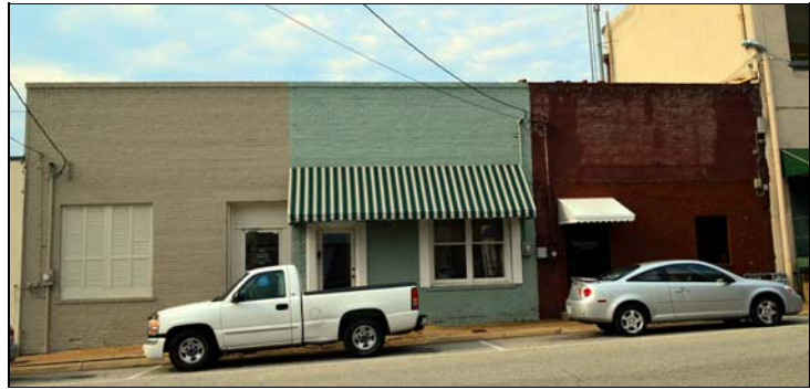
Figure 4.27. South elevation at buildings 13-10.03, 10.02, and 10.01 (left to right).
