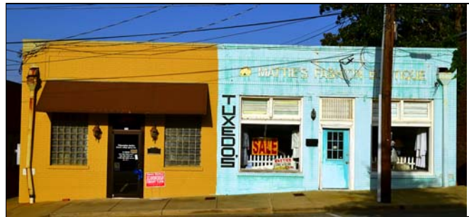
Figure 4.51. West elevation, building 9-49/9-48 (left to right).
