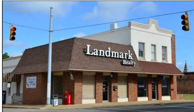
Figure 4.35. Landmark I and II, southeast oblique.
