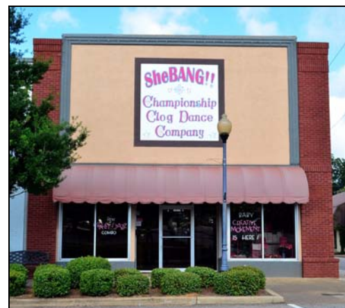
Figure 4.34. 13-63, SheBang, east elevation.
