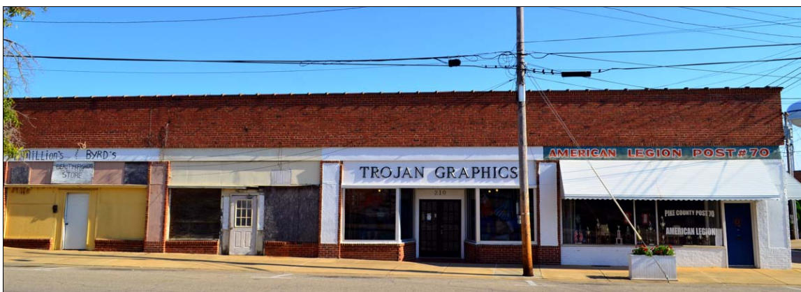
Figure 4.45. American Legion Building, south elevation.
