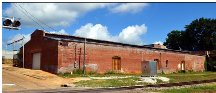
Figure 4.64. Henderson-Faulk Warehouse, southeast oblique.
