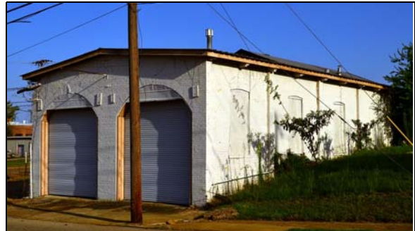
Figure 4.61. Troy Electric Pump House, northwest oblique.
