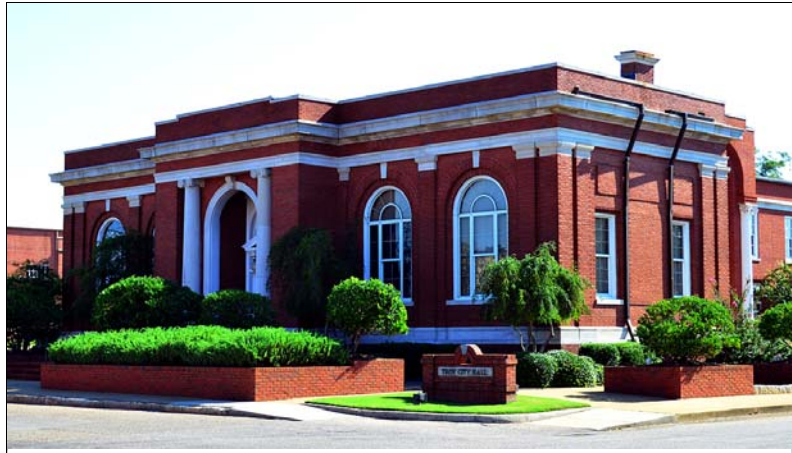
Figure 4.54. City Hall, southwest oblique.
